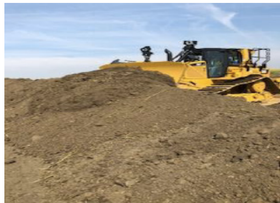
Men at work – km 195+620 – Aug 14, 2018
