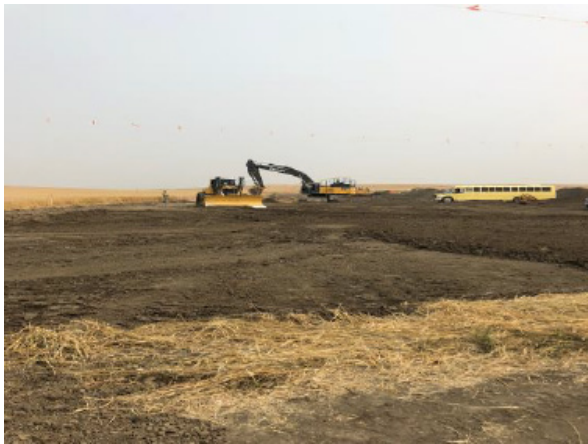
Dozer and excavator stripping – km 202+600 – Aug 16, 2018
