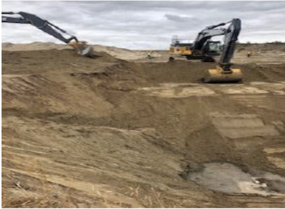
Bore pit and track bore machine – km 161+000 – Aug 13, 2018
