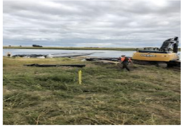
Aqua dam bags – km 165+100 -Aug 13, 2018
