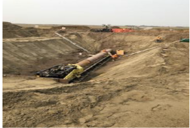
Track bore set up – km 161 + 000 – Aug 16, 2018
