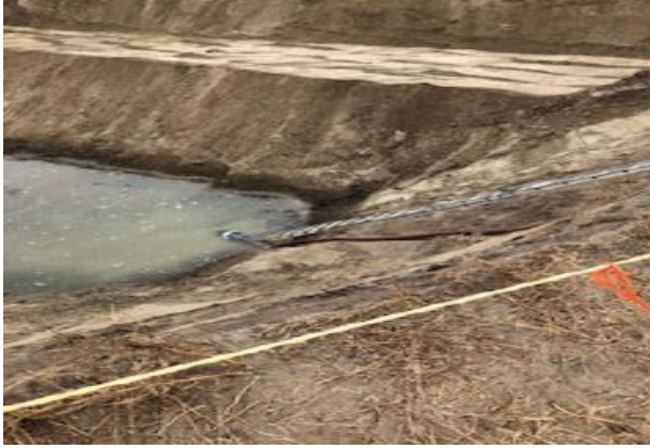
Bore hole pumping water – km 184+005 – Aug 15, 2018
