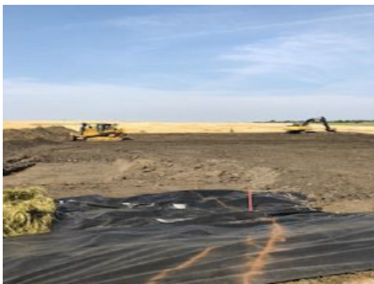
Stripping topsoil – SF 124 – Aug 14, 2018
