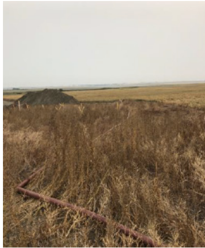
Pumping water - km 161+100 – Aug 15, 2018
