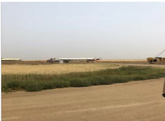
Side boom unloading wall – km 150+000 – Aug 17, 2018
