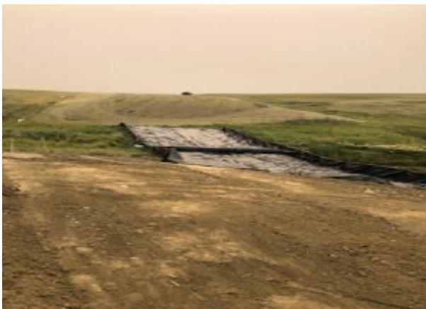
Access ramp before dirt put - Km 219+500 – Aug 15, 2018
