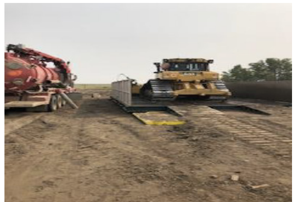
Dozer cleaning at wash station - 150+850 - Aug 17, 2018
