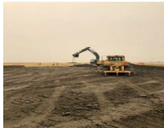
Ramp built over Sasktel lines– SF 124 – Aug 15, 2018
